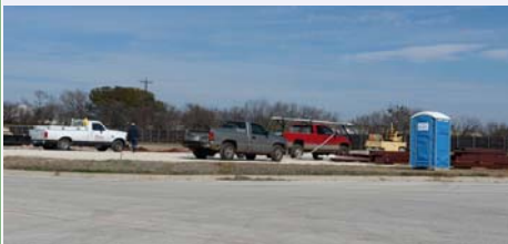
Work Begins on New Lab and Greenhouse Facilities
