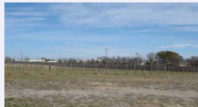
Trellis Installed, Irrigation System and Planting to be Completed this Spring
